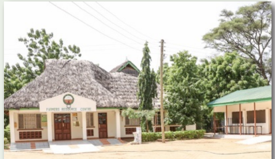
Turkana Sub-regional Research Centre
